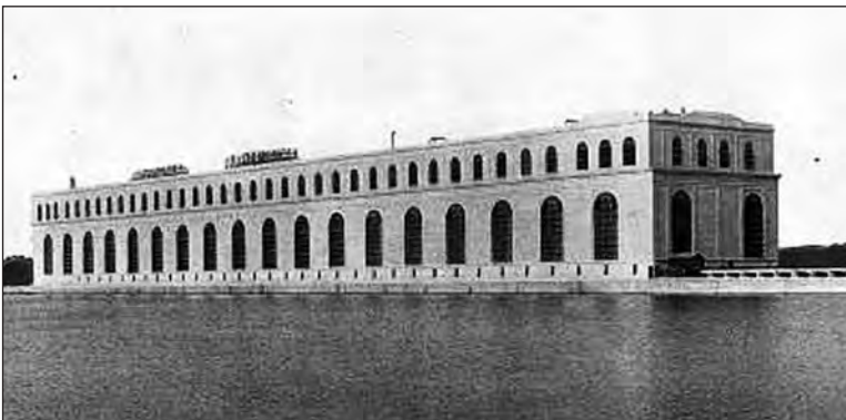
Fig. 7.7. Completed Keokuk Powerhouse
