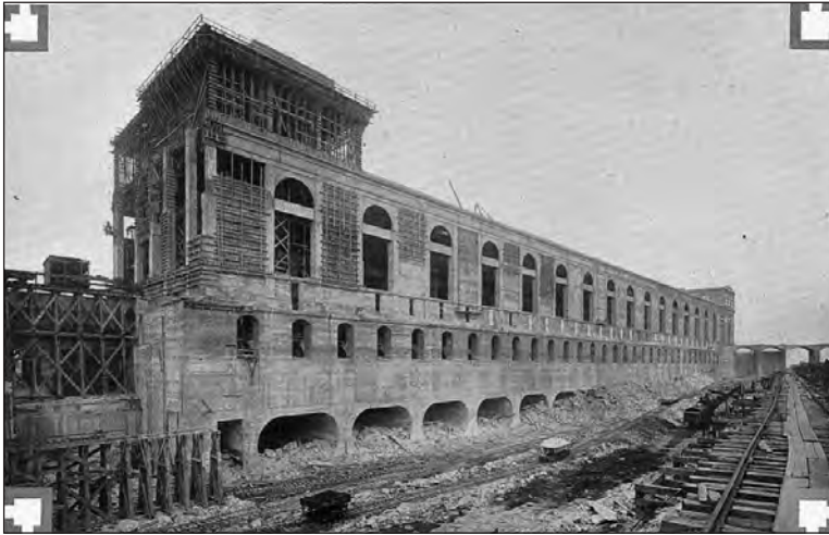
Fig. 7.6. Keokuk Powerhouse Construction
