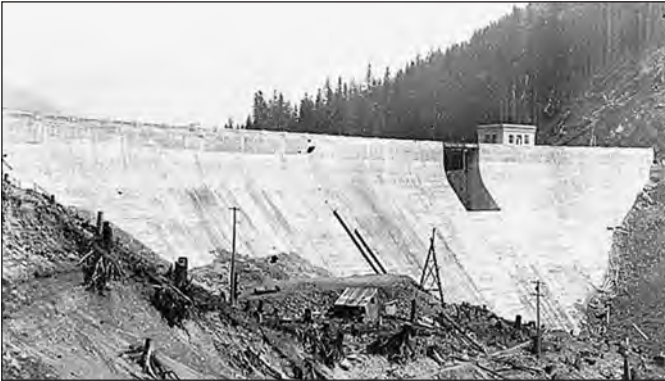
Fig. 10.7. Construction of Seattle City Light's Cedar River Dam Nearing Completion
