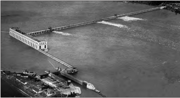
Fig. 7.2. Keokuk Dam and Powerhouse Panoramic View After Completion Lock and Drydock in Lower Foreground
