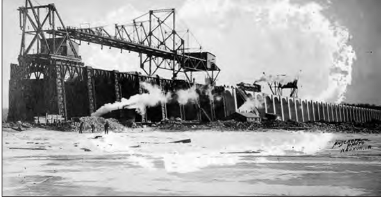
Fig. 7.4. Keokuk Main Dam Construction
