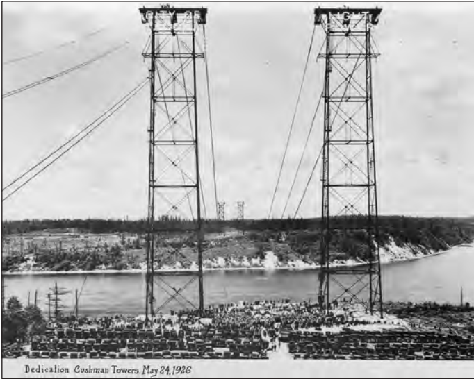
Fig. 10.9. Tacoma Power's Record-Setting 1.3 Mile Single-Span Transmission Line from Cushman No. 1
