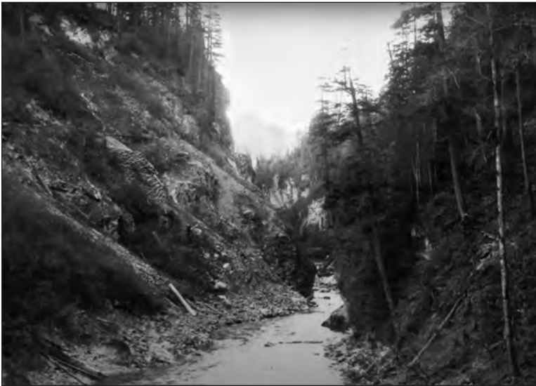
Fig. 10.10. Baker River Dam Site Before Construction Began
