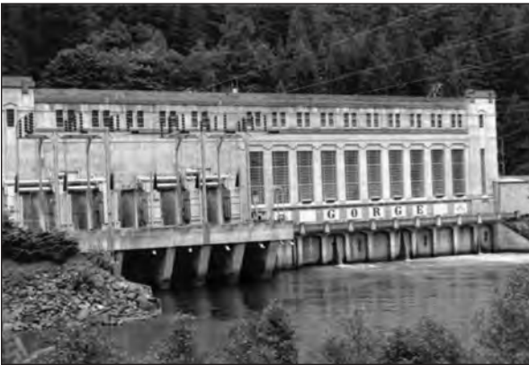
Fig. 10.6. Seattle City Light's Gorge Dam Powerhouse (left section added in the 1940s)
