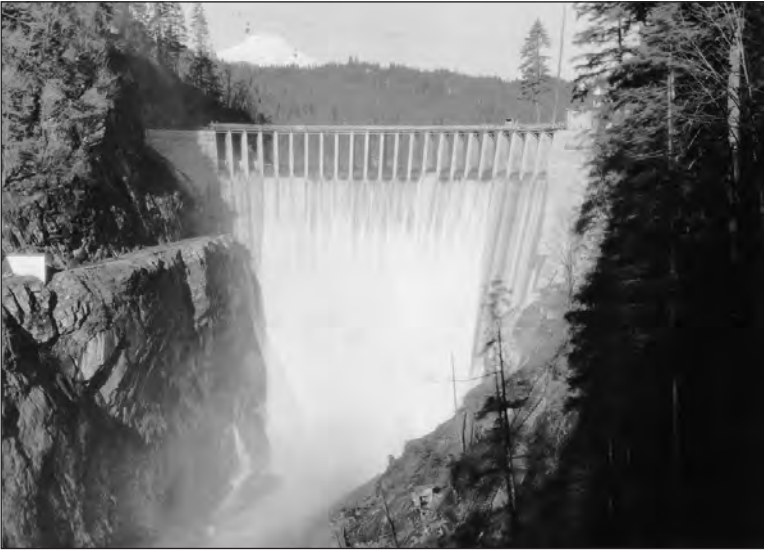
Fig. 10.11. Puget Sound Power & Light's Baker Dam
